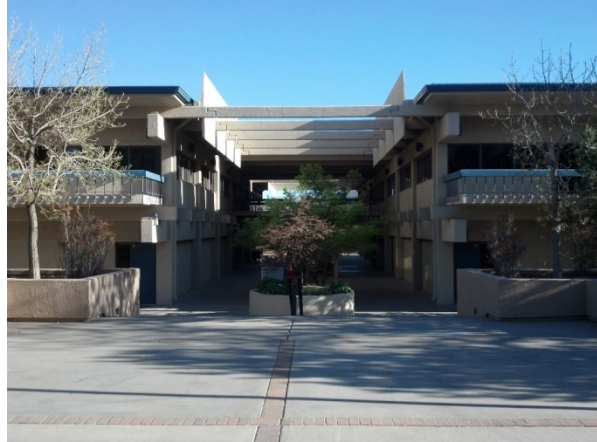
Anderson School (South entrance)
